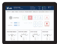
Monitoring and Local Control Screen
